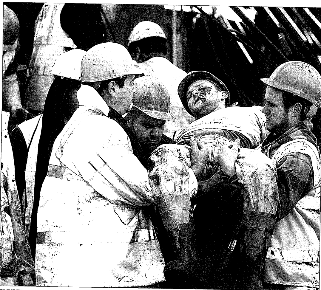
INJURED: a man is carried from the tangle of reinforcing bars, scaffolding and wet concrete
